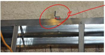
ROPERLY SIZED Z-clips WITH SPRAY FIREPROOFING HOWEVER, THE Z-CLIP SHOULD BE CUT DOWN THE Z-CLIP SHOULD TOP TRACK TO THE WIDH of the TOP TRACK TO THE WIDH of TRACK FOR PROPER DRYWALL OR FIRE FOR PROPER DRYWALL OR FIRE STOPPING INSTALLATION.
